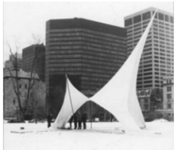
Figure 3: (a) Nylon-reinforced, double-curved ice structure with free edges
